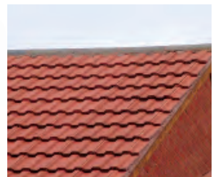
No chimney or flue
