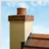
Brick or Stone Chimney (Class 1)
